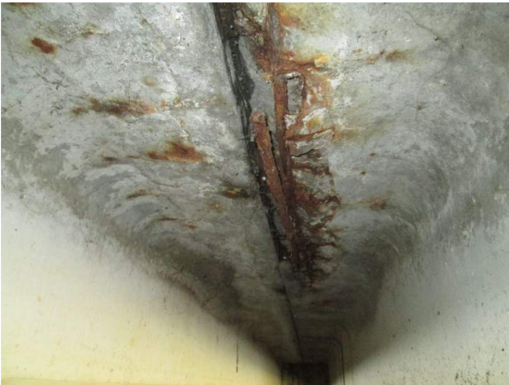
Underside of Deck at Joint 3
