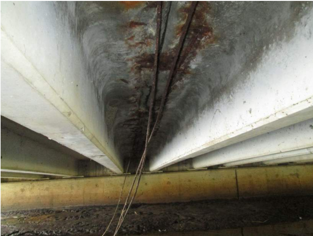
Underside of Deck at Joint 5 East
