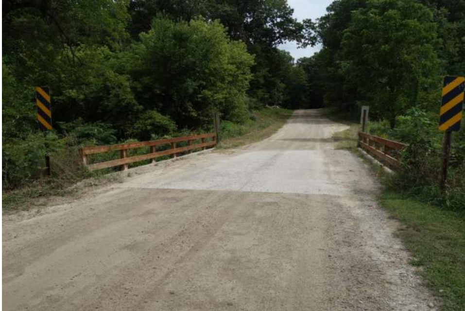
West Approach Looking East
