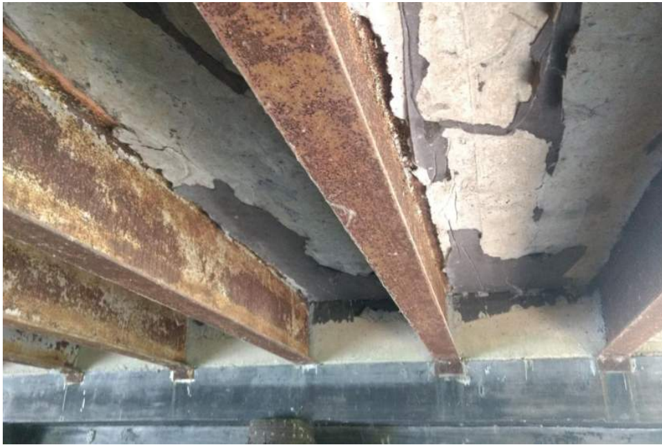
Typical Interior Beams and Deck Underside
