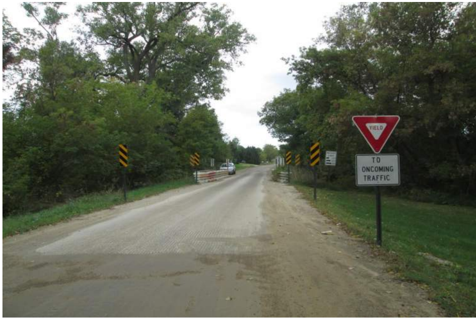
East Approach Looking West
