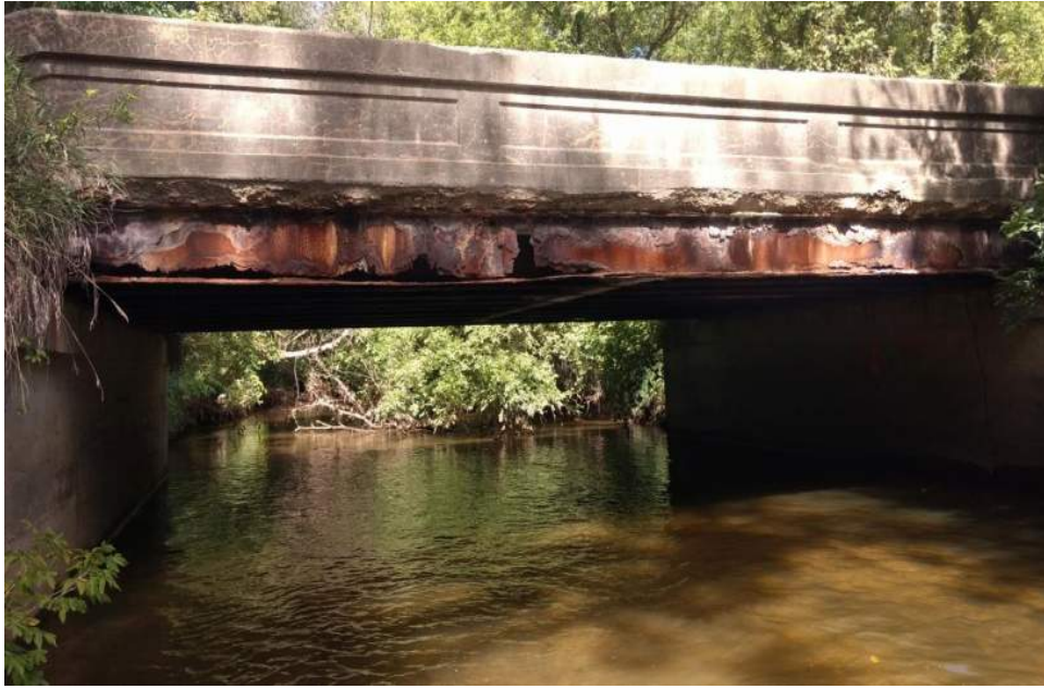
South Fascia Beam
