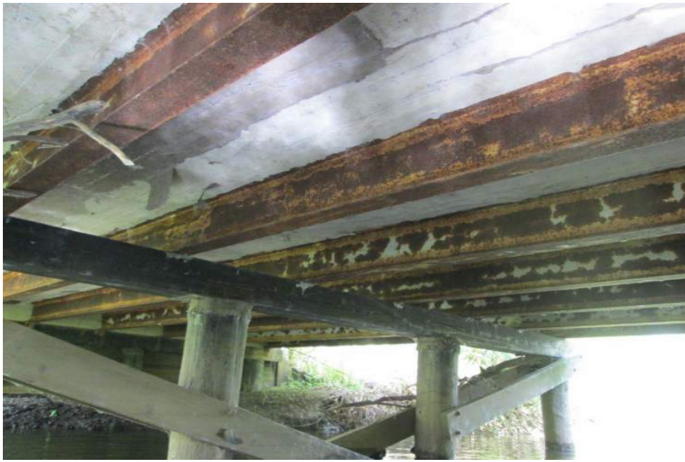
Typical Deck Underside
