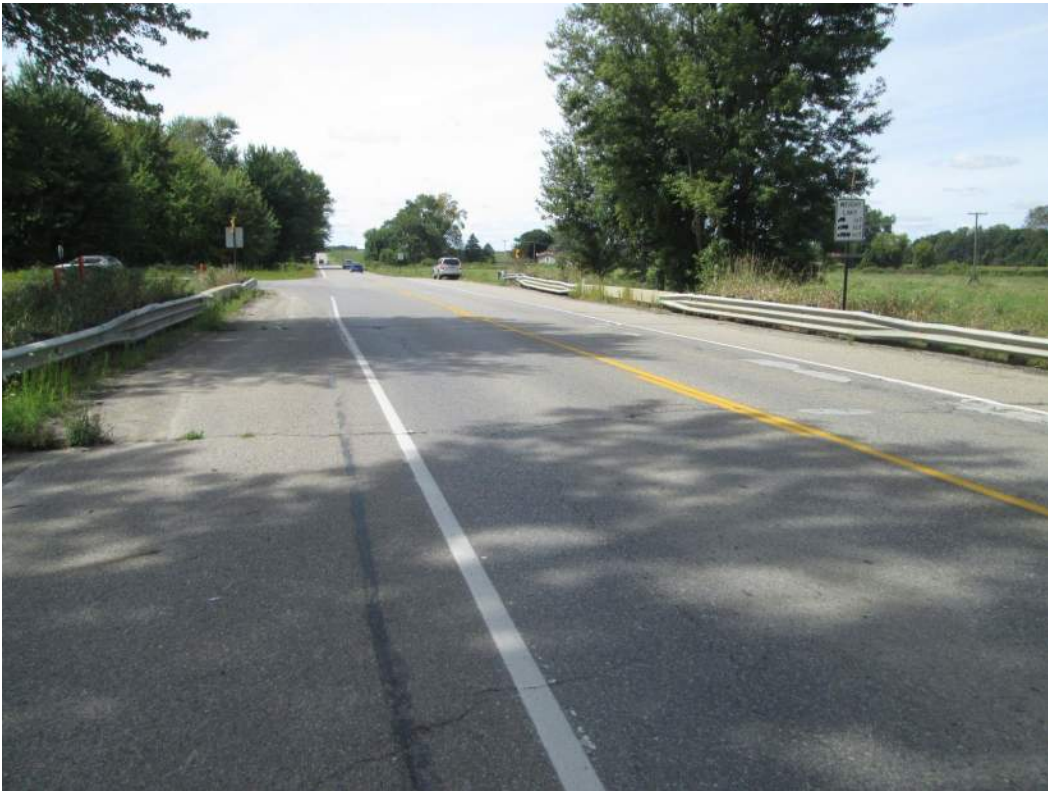
East Approach Looking West
