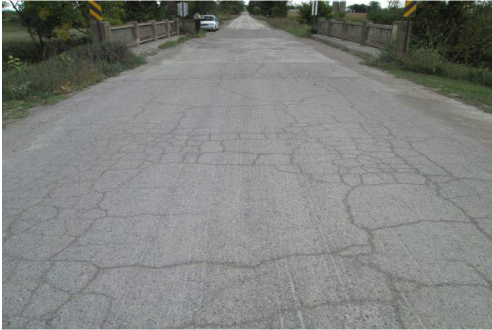
North approach looking south
