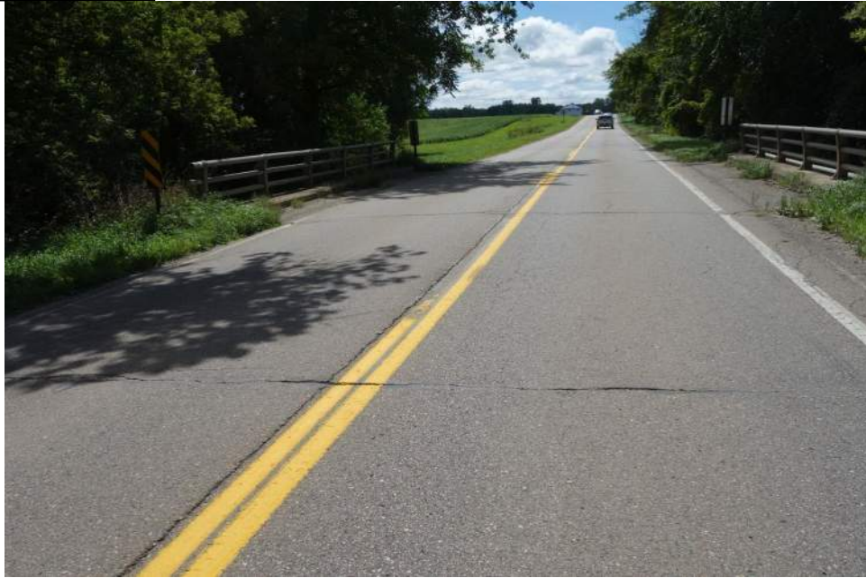
North Approach Looking South
