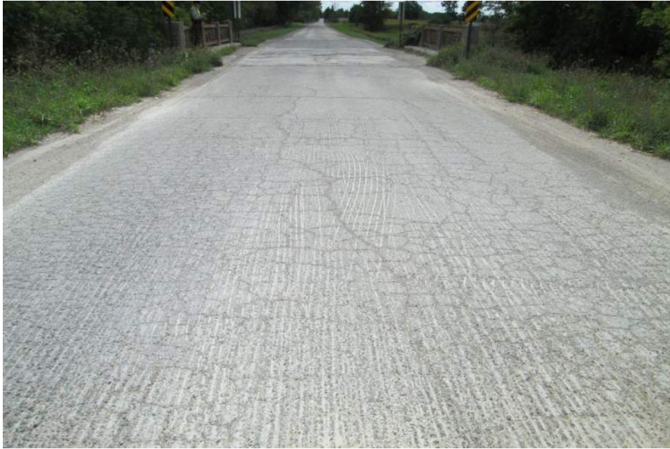
North approach looking south
