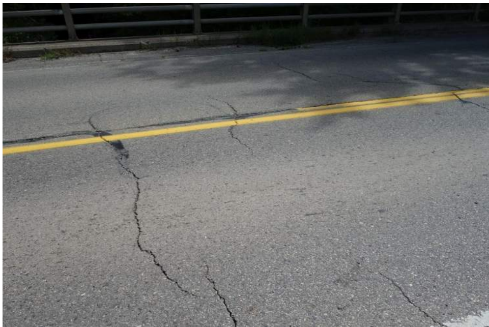
Typical Deck Surface
