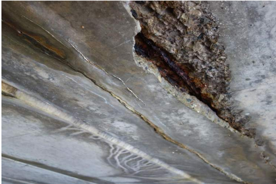
Beam 2W Exposed Steel
