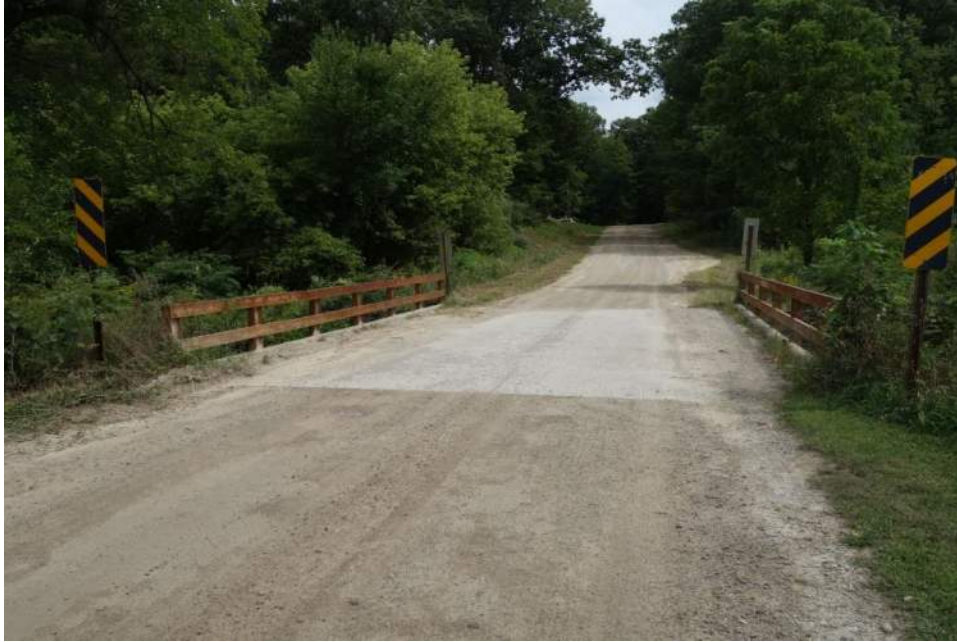
West Approach Looking East
