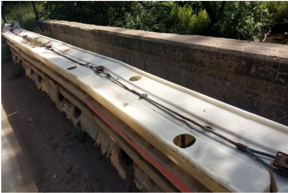
Typical Temporary Barrier
