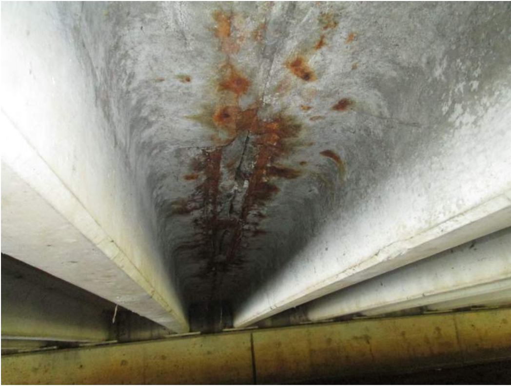
Underside of Deck at Joint 4
