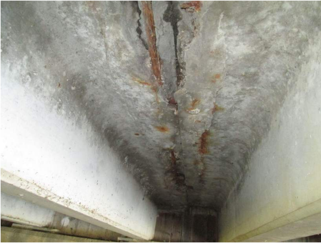
Underside of Deck at Joint 5 West
