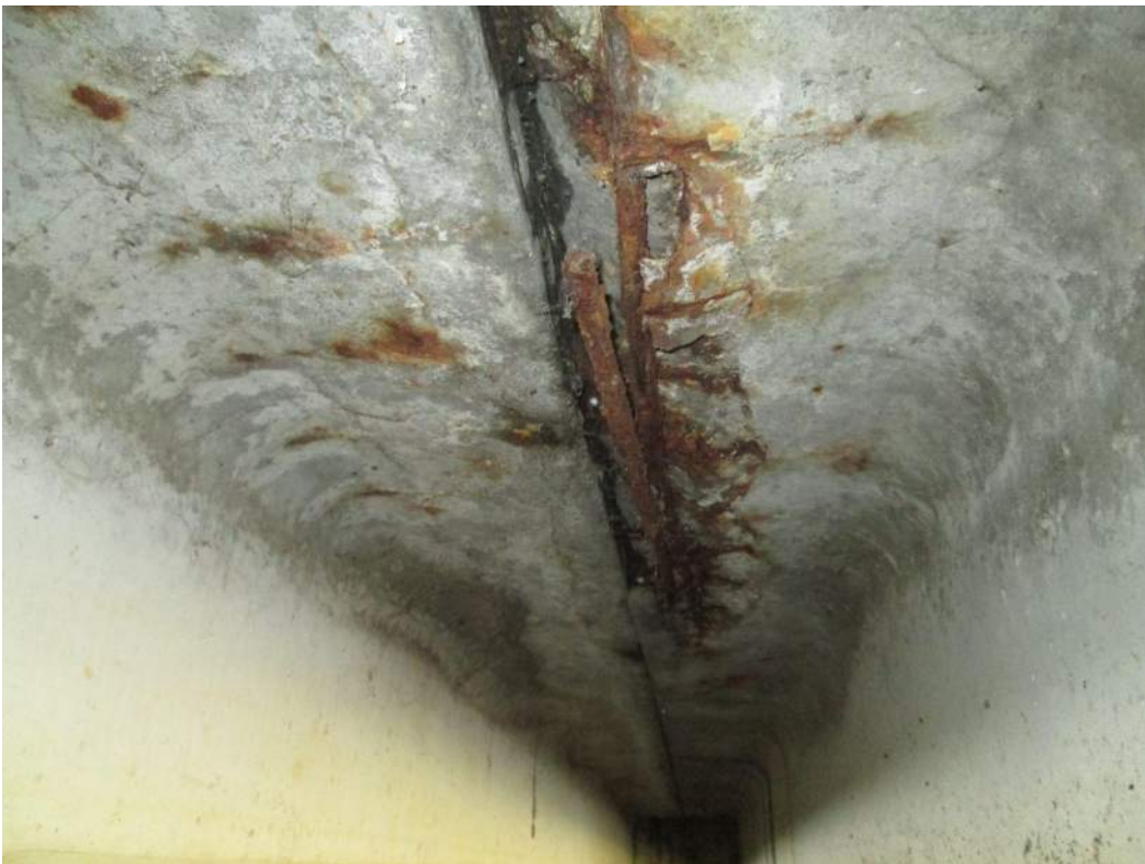
Underside of Deck at Joint 3
