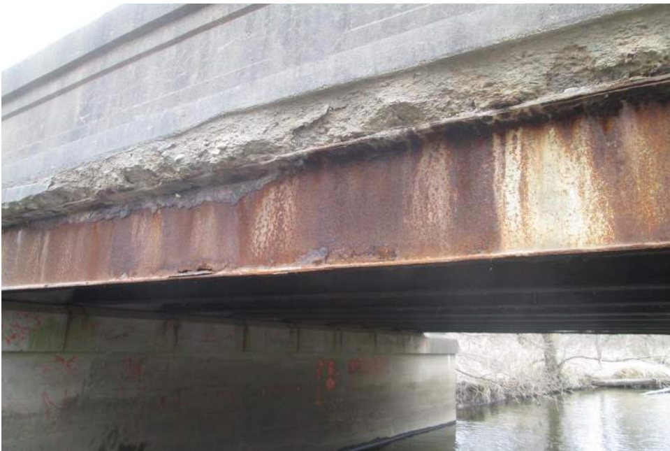
North Fascia Beam
